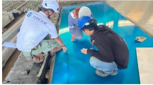
Gambar 3. 67 Proses pengecekan pipa sewage
