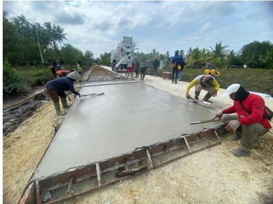
**Gambar 4. 14** Proses Finishing
