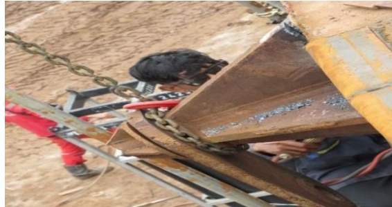
Gambar 4.13 transversal bulkhead
