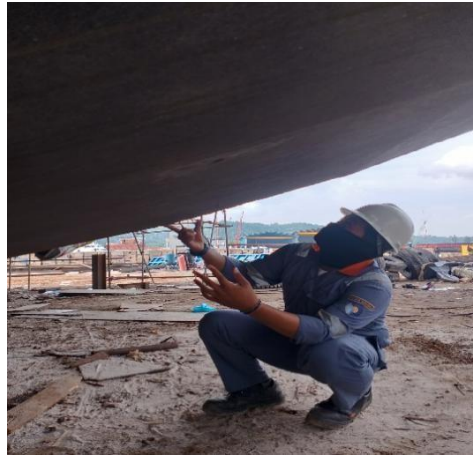
Gambar 3.10 Inspect welding panel main deck.
