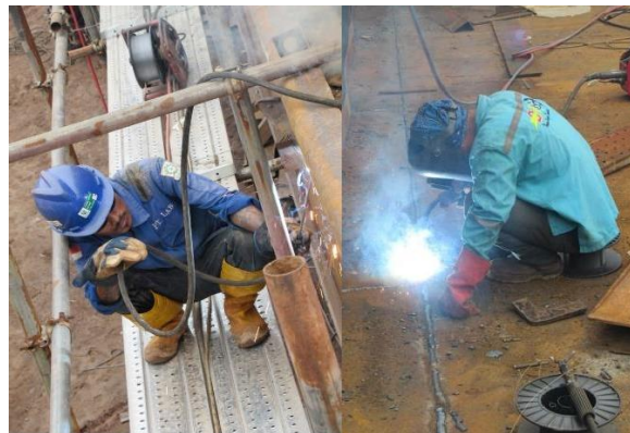
Gambar 4.16 welding blok Haluan
