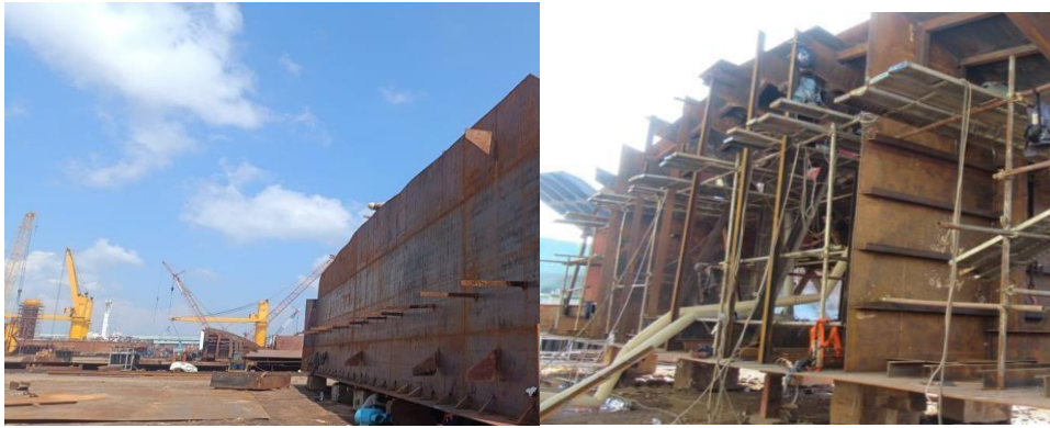
Gambar 4.12 transversal bulkhead
