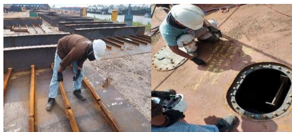
Gambar 3.26 welding inspection
