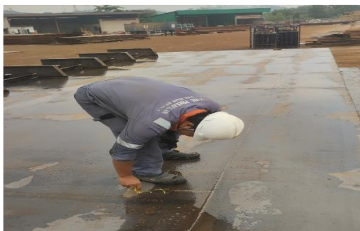
Gambar 3.40 inspect welding double bottom
