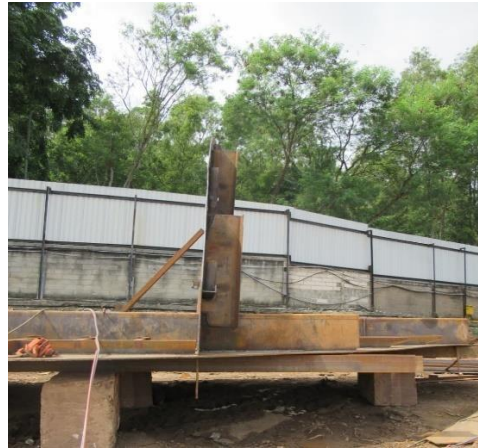
Gambar 4.9 Panel Main deck
