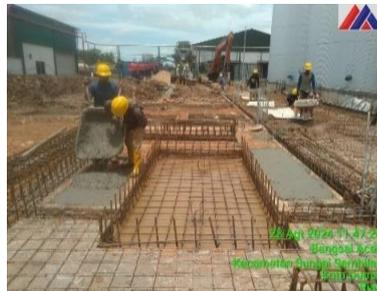
Gambar 3.39 Pemasangan Lean Concrete Slab Beton
