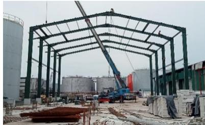
Gambar 3.59 *Erection CNP-50 Purlin*
