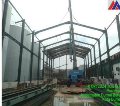
Gambar 3.58 *Erection WF 400 Rafter*
