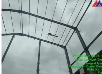
Gambar 3.60 *Erection Round Bar*
