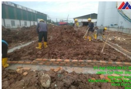
Gambar 3.36 Penimbunan Tanah Kembali Slab Beton
