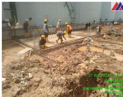
Gambar 3.34 Pemasangan *Rebar Ground Beam*
