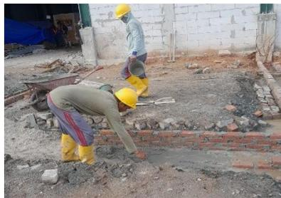
Gambar 3.32 Pemasangan *Lean Concrete Ground Beam*
