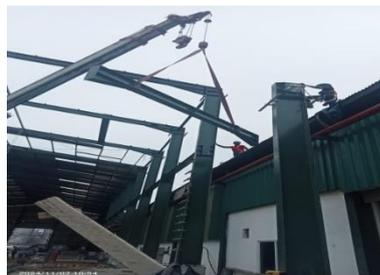
Gambar 3.57 *Erection* WF-200 Beam
