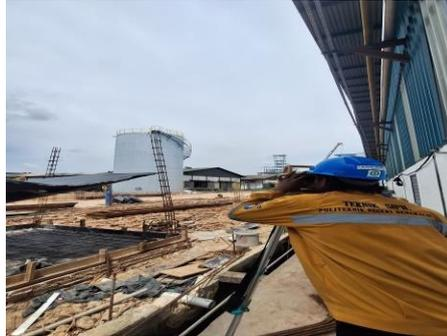
Gambar 3. 19 Pekerjaan Penentuan as *pile cap*
