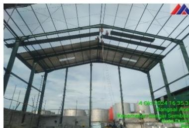
Gambar 3.63 Instal Aluminium Foil
