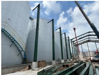
Gambar 3.56 *Erection* WF 500 Colum
