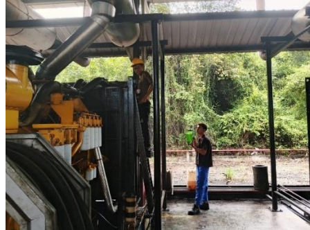
Gambar3. 58 Proses pengisian air radiator
