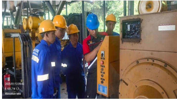
Gambar 3. 1 Praktik Pengoperasian Panel Genset.
