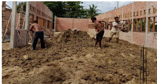
Gambar 3. 52 Penimbunan Tanah
