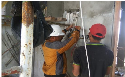
Gambar 3. 71 Instalsi Stop Kontak
