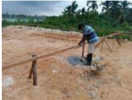
Gambar 3. 81 Bowplank galian pondasi
