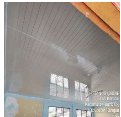
(c) Gedung C
