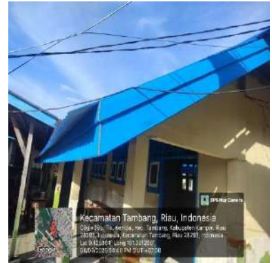
(c) Gedung C
