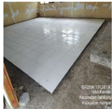
(c) Gedung C
