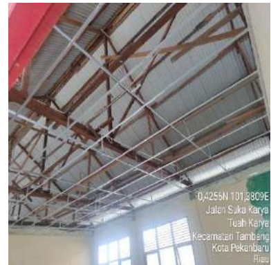
(c) Gedung C
