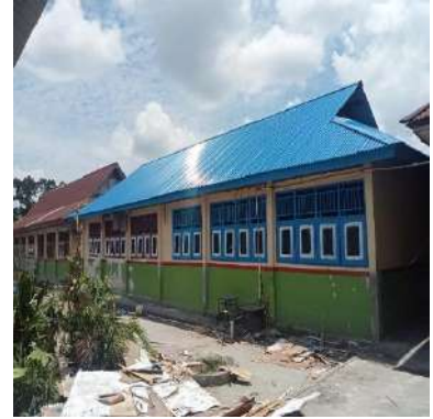
(c) Gedung C
