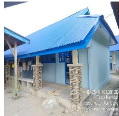
(c) Gedung C
