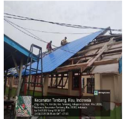
(c) Gedung C
