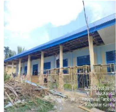
(c) Gedung C
