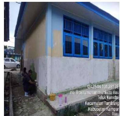
(c) Gedung C
