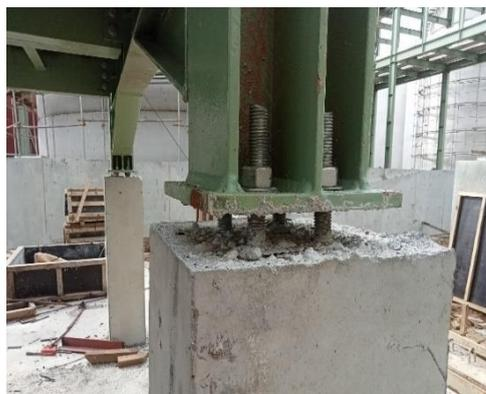
*Gambar 3.5 Cutting kolom pedestal*
