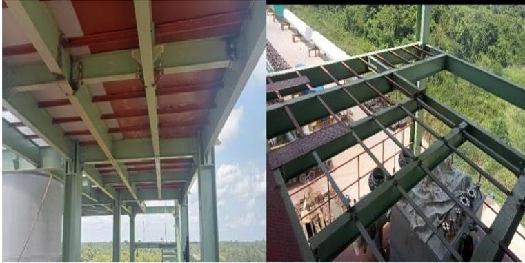
44. (Rabu, 11 September 2024) Erection gording dan bracing atap.
