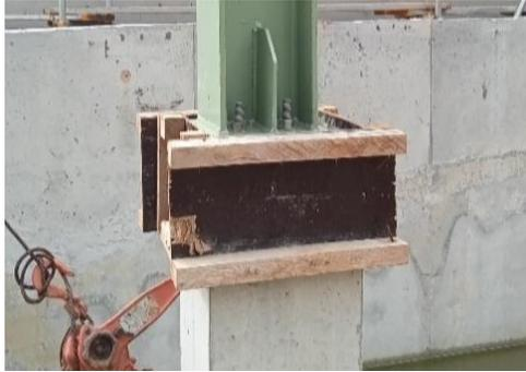
Gambar 3.6 Proses Grouting kolom pedestal
