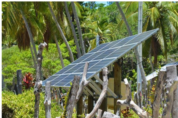
Gambar 3.5 Instalasi Solar Panel
