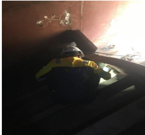
Gambar 3. 47 Marking Visual Welding Inspection Sumber : Penulis
