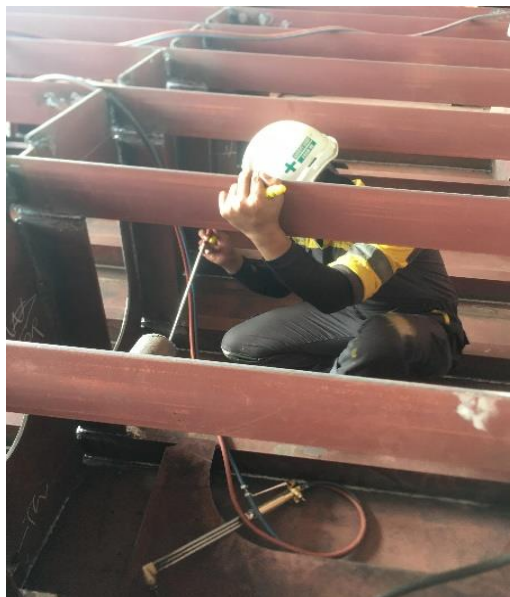
Gambar 3. 54 Marking Visual Welding Inspection Sumber : Penulis
