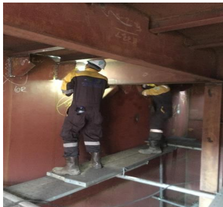
Gambar 3. 56 Marking Visual Welding Inspection Sumber : Penulis
