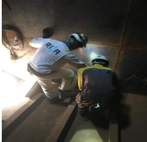
Gambar 3. 61 Marking Visual Welding Inspection Sumber : Penulis
