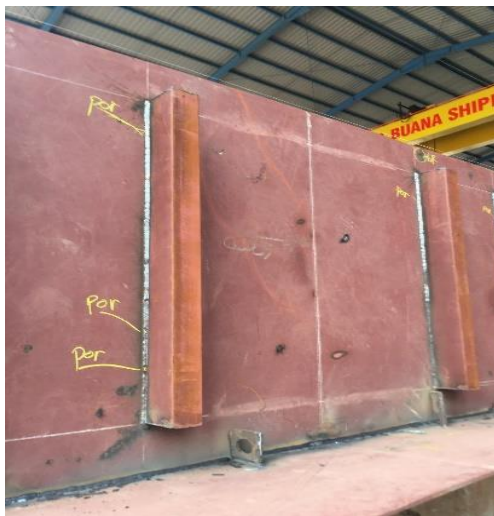
Gambar 3. 60 Marking Visual Welding Inspection Sumber : Penulis
