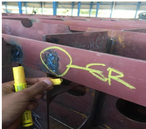
Gambar 3. 57 Marking Visual Welding Inspection Sumber : Penulis
