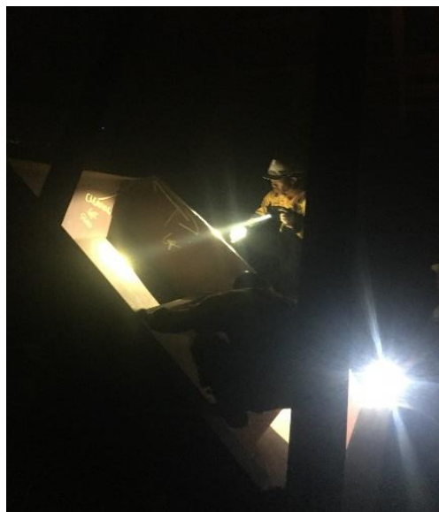
Gambar 3. 40 Marking Visual Welding Inspection
