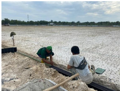
Gambar 3. 18 Pekerjaan ex. aquatech sport
