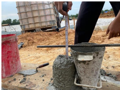
Gambar 3. 29 Uji slump beton ready mix K-225
