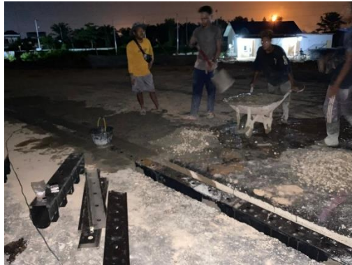
Gambar 3. 19 Pekerjaan ex. slotted channel
