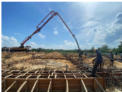
Gambar 3. 53 Pengecoran slump sloof
