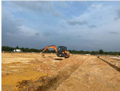
Gambar 3. 9 Pengalian pipa HDPE
