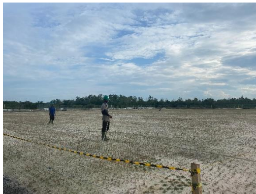
Gambar 3. 15 Perawatan rumput Zoysia Matrella
