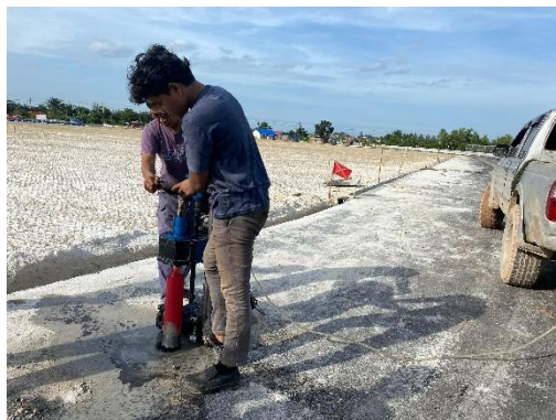
Gambar 3. 36 Core drill aspal
