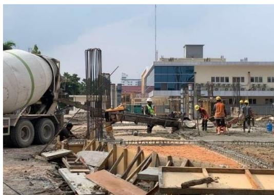
Gambar 2 3 Beton Ready Mix
