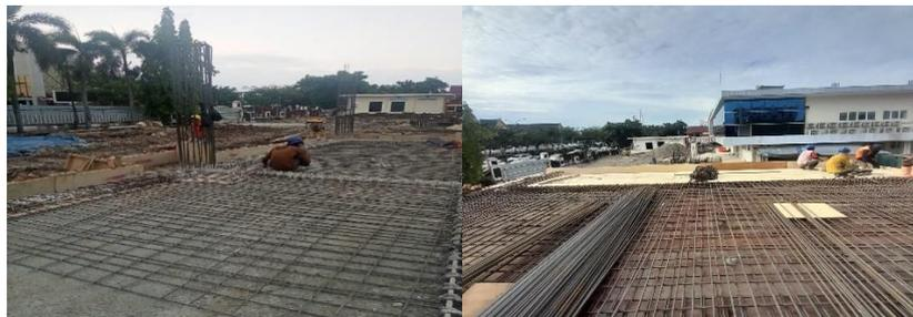
Gambar 3. 27 Pemasangan Wiremesh
