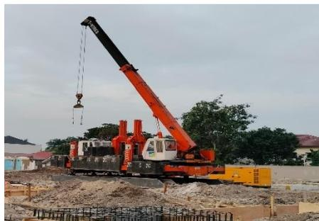
Gambar 2 10 HSPD (Hidrolic Static Pile Driver)
