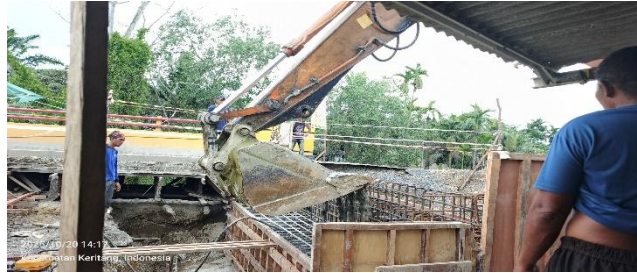
Gambar 3.36 Pengecoran Abutment
