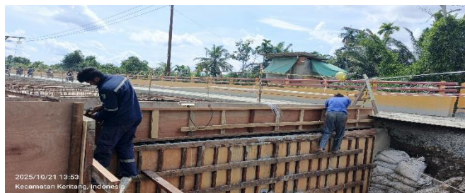
Gambar 3.37 Pembongkaran Bekisting Abutment
