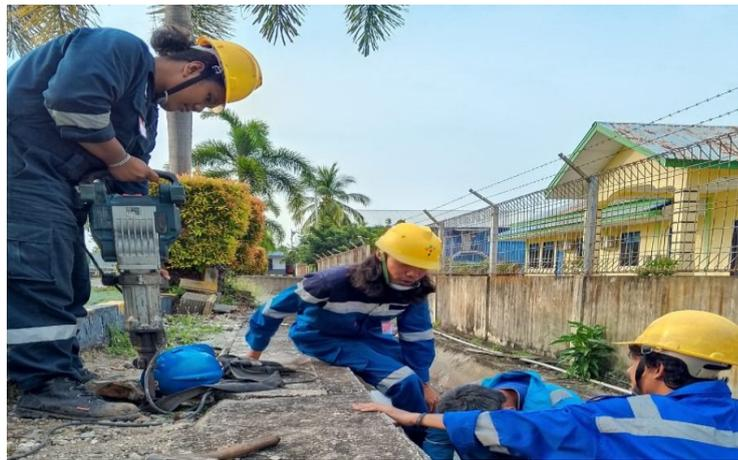
Gambar 3.5 penggantian line pipa air 2 inch
