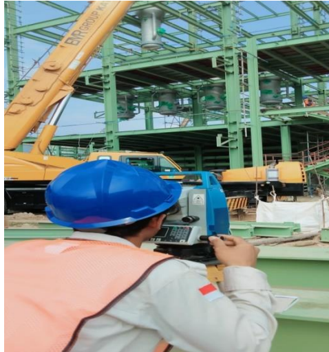
Gambar 3.11 verticality kolom
