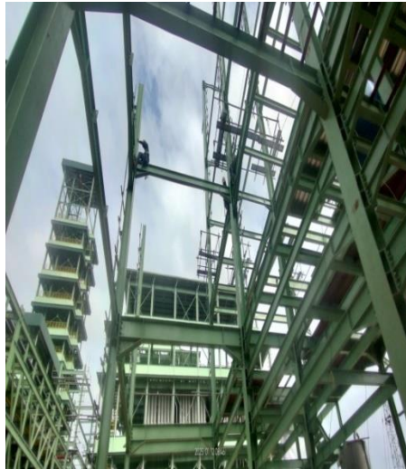
Gambar 3.9 erection secondary beam lengkapi baut
