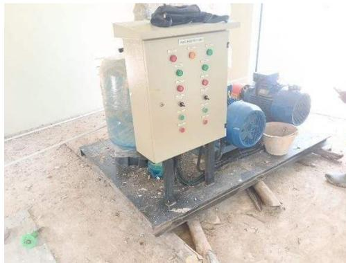
Gambar 3.75 Pompa Siram Rumput *Type Centrifugal*
