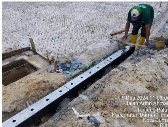
Gambar 3.79 Pemasangan ex. *Slloted channel*
