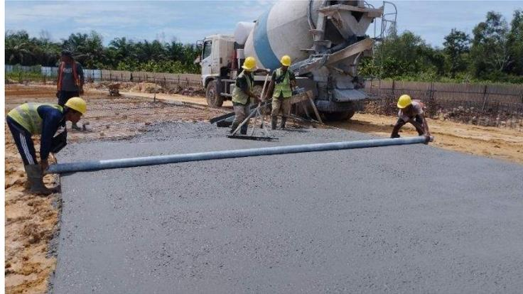
Gambar 3.85 Cor Beton K-225
