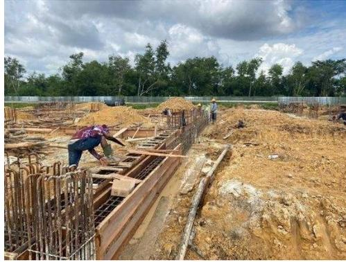
Gambar 3.60 Instal Bekisting Sloof
