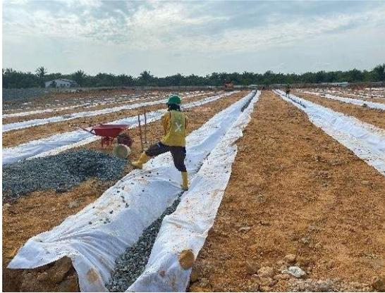
Gambar 3.66 Pegadaan Pipa HDPE *Perforated Corrugated* Dia 4 (
