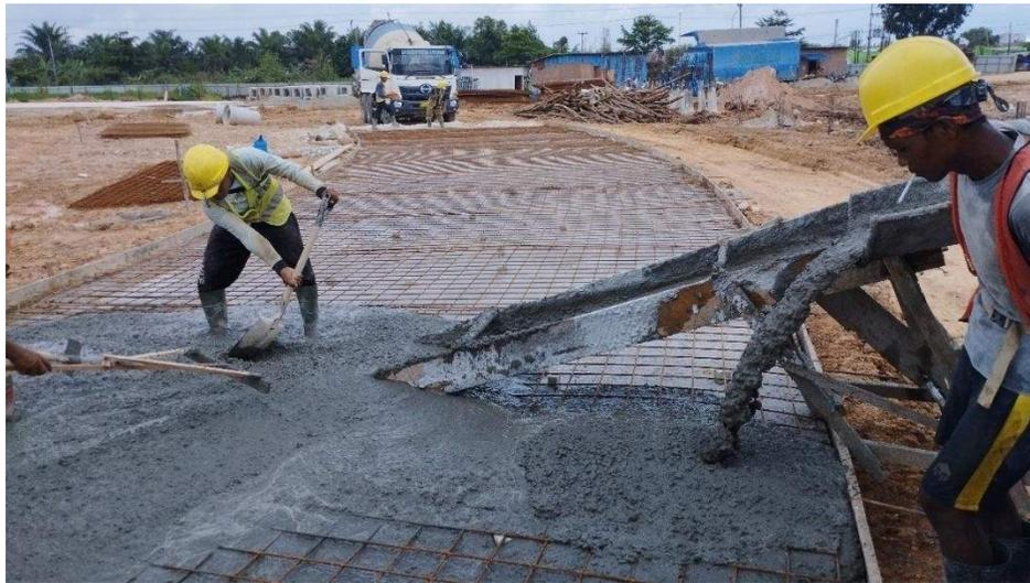
Gambar 3.120 proses beton dialirkan
