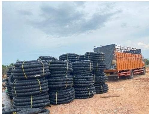
Gambar 3.67 Pegadaan Pipa HDPE *Perforated Corrugated* Dia 4
