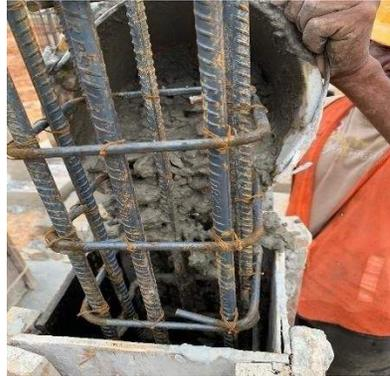
Gambar 3.19 Penuangan Beton Kedalam Bekisting
