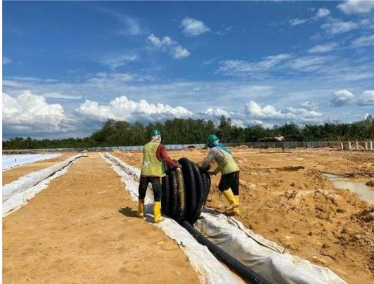
Gambar 3.68 Instalasi Pipa HDPE *Perforated Corrugated* Dia 4
