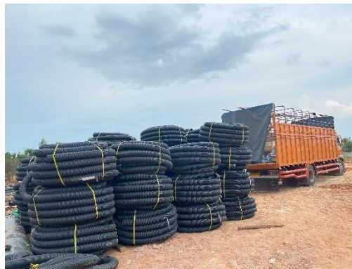
Gambar 3.67 Pegadaan Pipa HDPE Perforated Corrugated Dia 4 ( Sumber: Dokumentasi Lapangan, 2024 )
