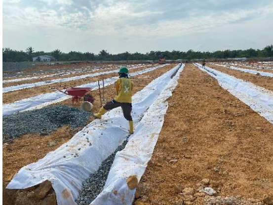
Gambar 3.66 Pegadaan Pipa HDPE Perforated Corrugated Dia 4 ( Sumber: Dokumentasi Lapangan, 2024 )
