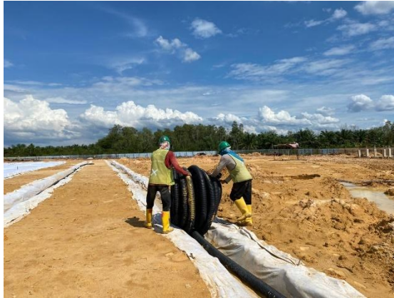
Gambar 3.68 Instalasi Pipa HDPE Perforated Corrugated Dia 4 ( Sumber: Dokumentasi Lapangan, 2024)
