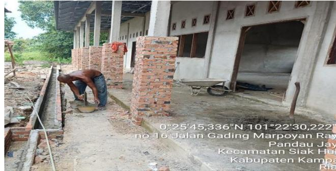
Gambar 3. 24 Plasteran Kolom Teras
