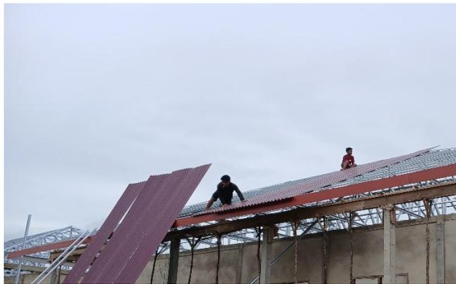
Gambar 3. 45 Pemasangan Atap Long Spandek
