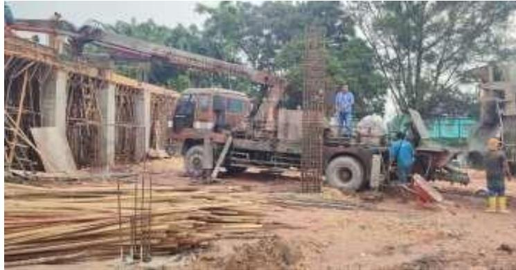
Gambar 3. 45 Concrete Pump
