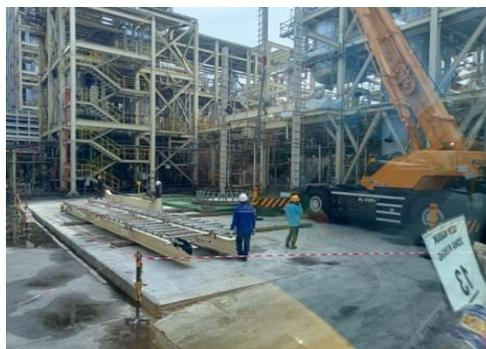
Gambar 3.37 Proses Erection Kolom
