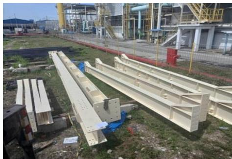
Gambar 3.36 Proses *Finishing*
