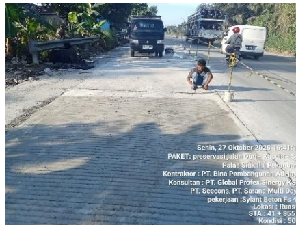
Gambar 3. 53 joint sealant (Sumber Dokumentasi Lapangan 2025)
