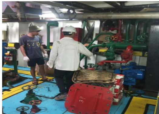
Gambar 3. 38 Proses Pengecekan Hasil Repair
