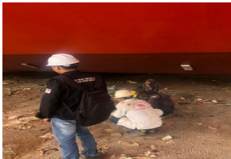
Gambar 3. 31 Proses Air Test
