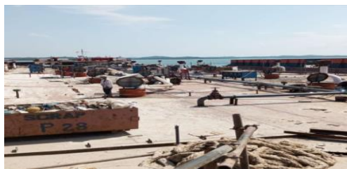
Gambar 3. 8 Repair Oil Barge bagian Deck
