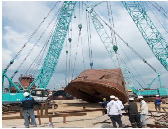
Gambar 3. 18 Proses Turning Blok
