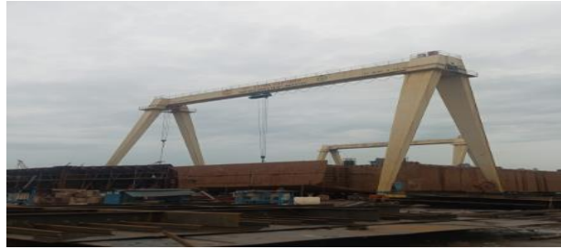
Gambar 2.11 . Overhead Crane kapasitas 25 ton
