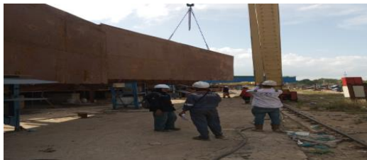
Gambar 3. 7 Proses Erection Shed Shell
