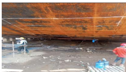
Gambar 3. 26 Proses Repleting Plat
