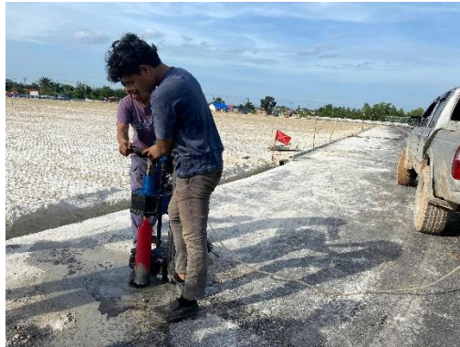
Gambar 3. 36. Core drill aspal
