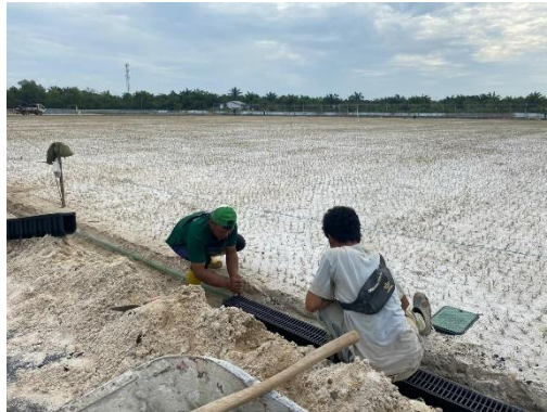
Gambar 3. 18. Pekerjaan ex. aquatech sport
