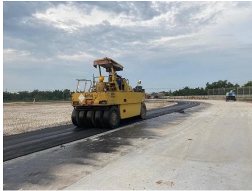
Gambar 3. 34. Pengilasan lapisan aspal AC-WC
