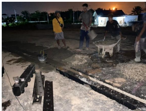
Gambar 3. 19. Pekerjaan ex. slotted channel
