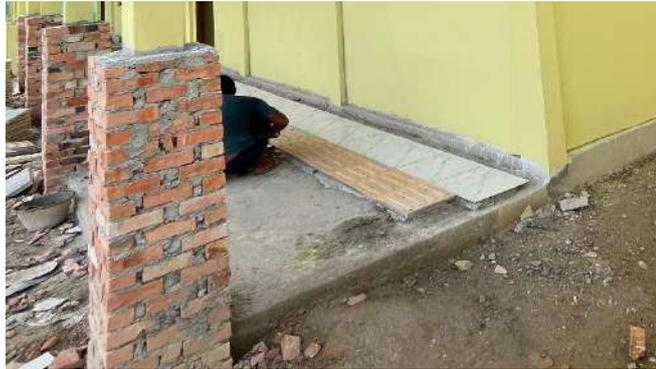
Gambar 3. 39 Pemasangan Block Dan Warning Block
