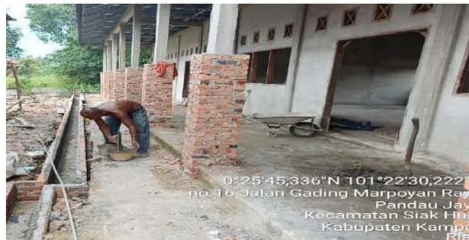
Gambar 3. 24 Plasteran Kolom Teras
