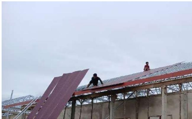
Gambar 3. 45 Pemasangan Atap Long Spandek
