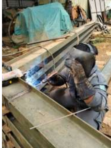
Gambar 3. 28 Pengelasan Besi H Beam
