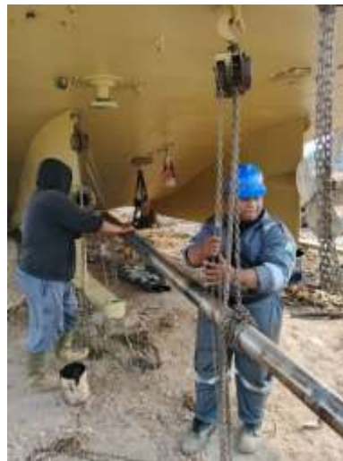
Gambar 3. 7 Pemasangan As Propeller
