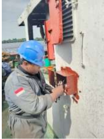
Gambar 3. 14 Memasang Tali Shut-Off Valve
