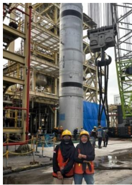
Gambar 3. 46 Lifting Vessels Reactor
