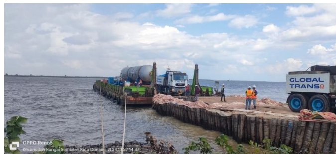
Gambar 3. 42 Pemindahan Vessels Reactor
