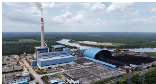
Gambar 1. 1 PT PLN NUSANTARA POWER UP TENAYAN
