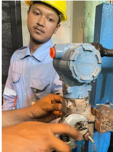
Gambar 2. 3 Kalibrasi Pressure Transmitter
