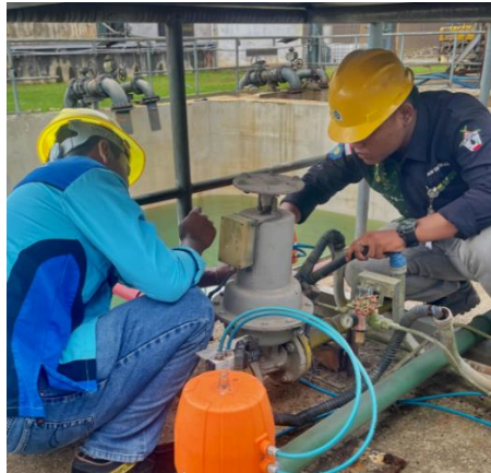
Gambar 2. 9 Pengantian Selenoid Valve
