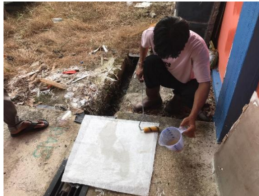
Gambar 4. 5 Proses Laminasi
