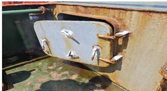
Gambar 4.10 Proses Pemarkingan Togel Hatch Cover Steering Room
