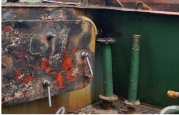
Gambar 4.62 Hasil Pekerjaan Pergantian Togel Hatch Cover Stearing Room
