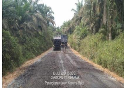
( Gambar 3. 12 Asphalt Sprayer)
