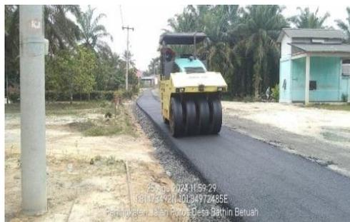
(Gambar 3. 10 Pneumatic Tired Roller)
