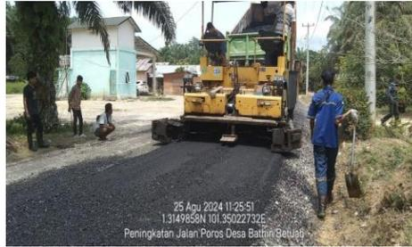
(Gambar 3. 9 Asphalt Finisher)
