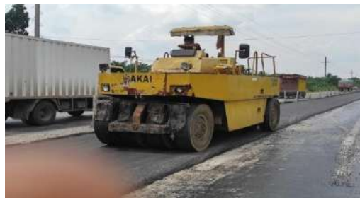
Gambar 3. 8 Alat berat Pneumatic Tier Roller
