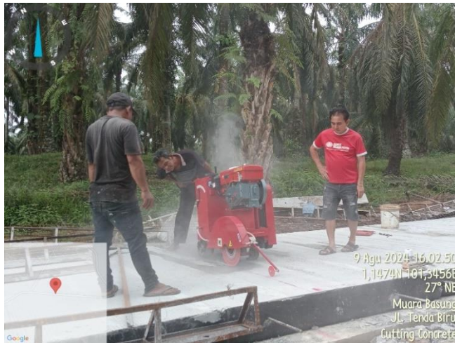
Gambar 4.22 (Cutting Concrete) Sumber : Dokumentasi Lapangan, 2024
