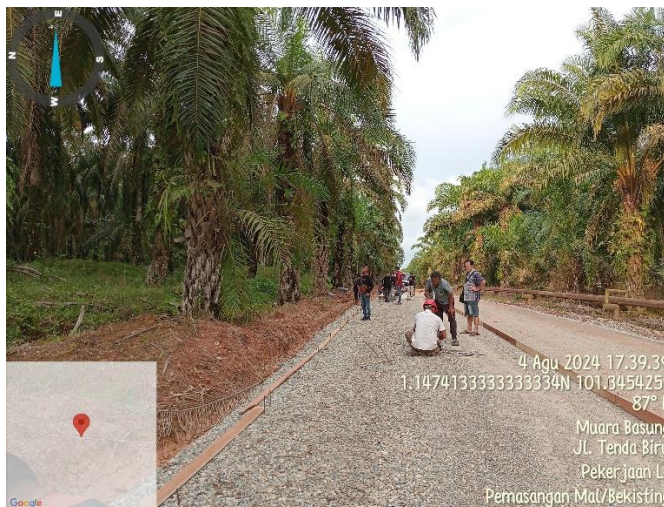
Gambar 3.15 (Pemasangan Mal/Bekisting LC)
