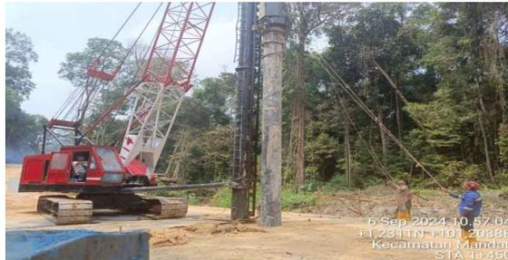
**Gambar 3.5** Diesel Hammer
