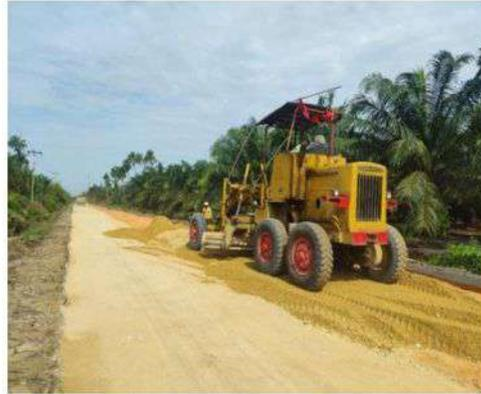
**Gambar 3. 4 Motor Grader**
