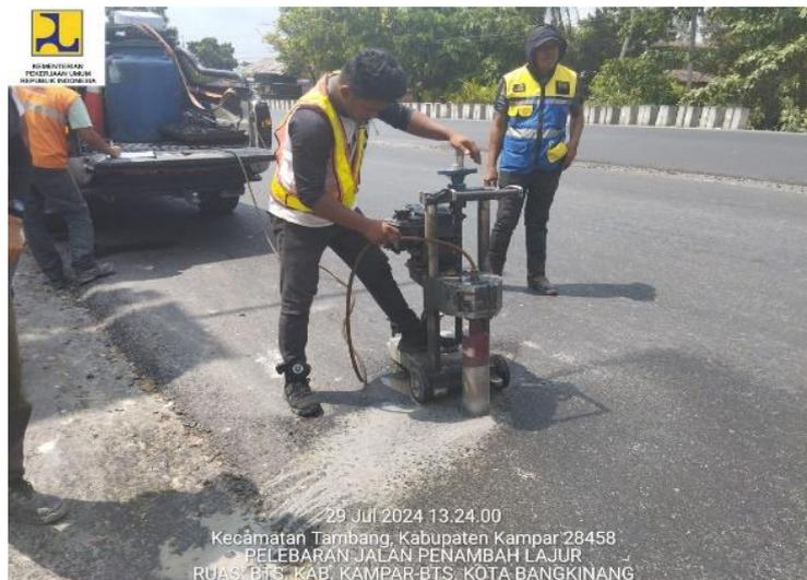
**Gambar 3.15 Core Drill Aspal**
