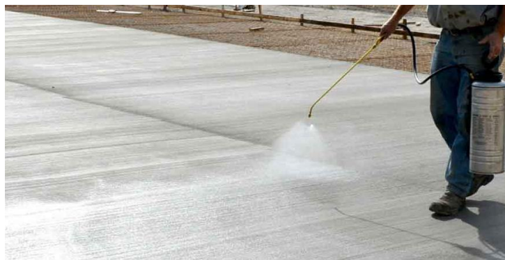
Gambar 4. 9 Curing Compound sumber: pekerjaan dilapangan
