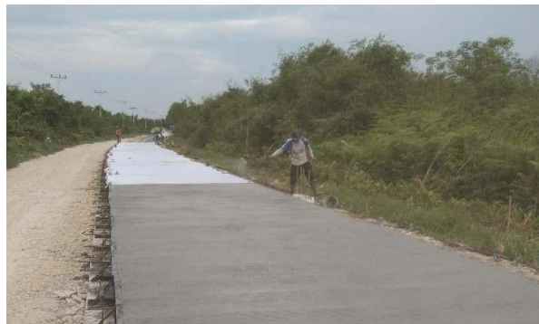
Gambar 3. 25 Pekerjaan Curing Compound
