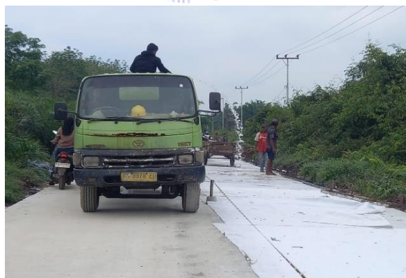
Gambar 3. 26 Perawatan Curing
