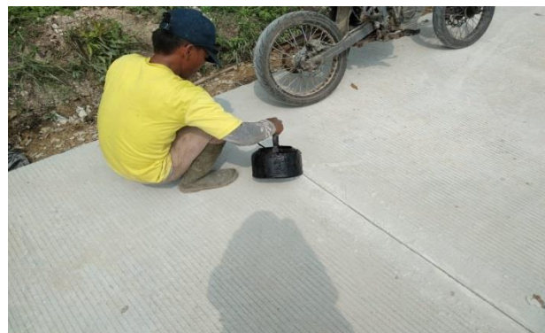
Gambar 3. 28 Pekerjaan Joint Sealing
