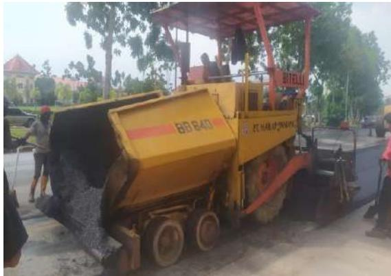
Gambar 4.5. Asphalt Finisher
