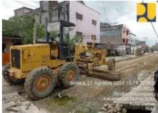
Gambar 3. 17 Motor Grader
