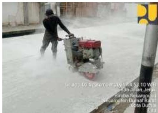
Gambar 3. 21 Mesin Cutting
