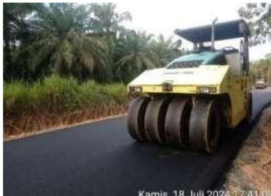
*Gambar 3.6 Pneumatic Tire Roller
