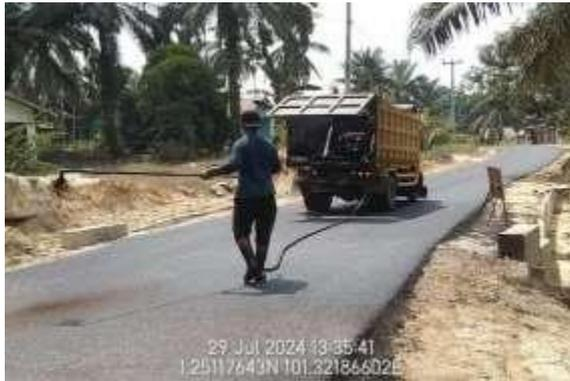
Gambar 3. 3 Asphalt Distributor
