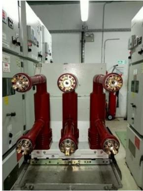
Gambar 4. 1 Vacuum circuit breaker
