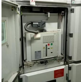
Gambar 4.4 VCB (*Vacuum Circuit Breaker*)
