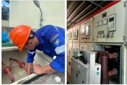
Gambar 3.1 VCB (Vacuum Circuit Breaker)
