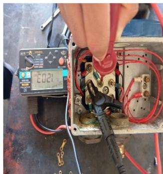
Gambar 4.3 *Resistansi Test Phase To Phase*
