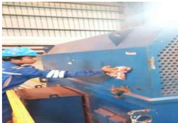
Gambar 3. 45 preventive maintenance motor cooling tower unit 2
