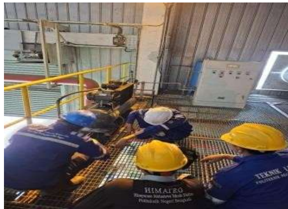
Gambar 3. 39 pengetesan compresor BusDuct Unit 2
