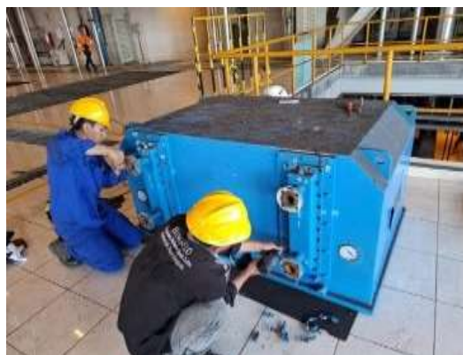
Gambar 3. 70 progres repair cooler motor Boiler Feed Pump
