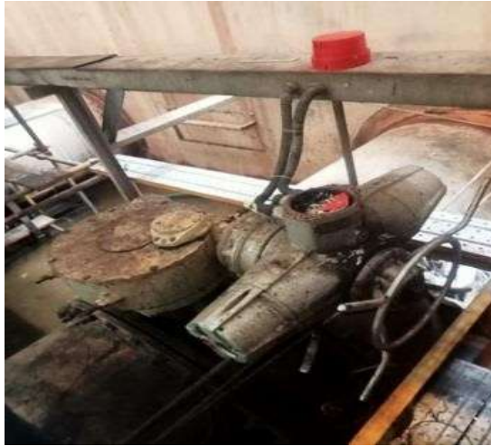
Gambar 3. 63 penormalan motor operated valve (MOV)
