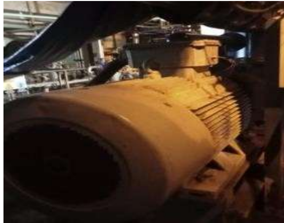
Gambar 3. 26 pengecekan Motor Ex Close Cycle Water Pump
