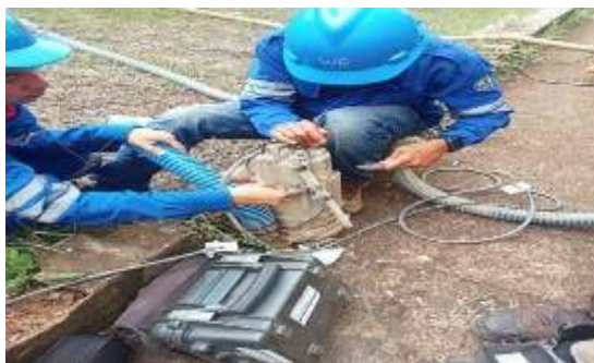
Gambar 3. 52 connect sumppump di area WTP
