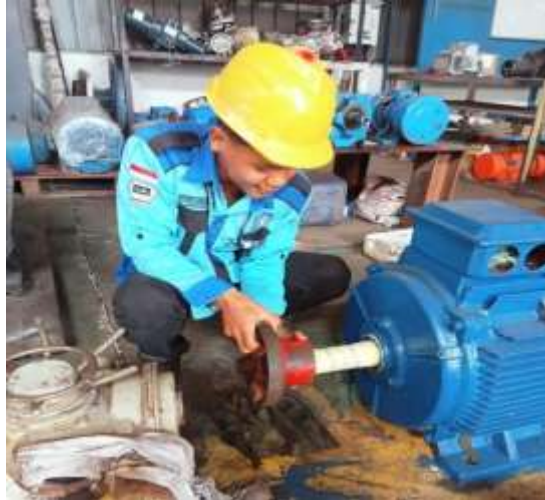
Gambar 3. 102 Gambar penggantian bearing motor
