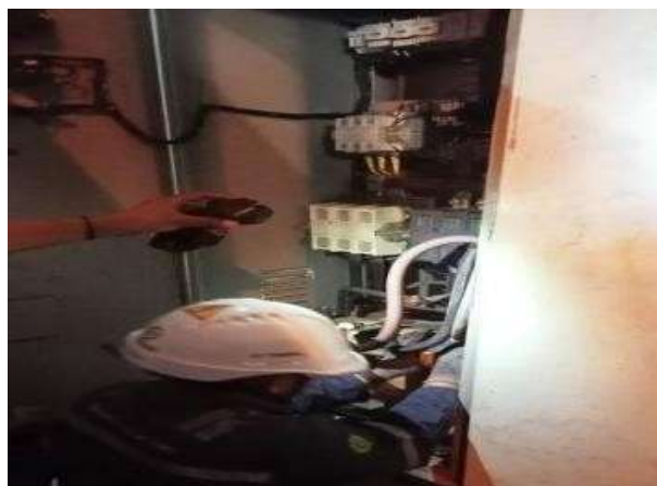
Gambar 3. 19 pengecekan panel hospot GT 4
