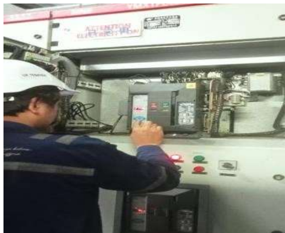
Gambar 3. 15 load test breaker C01 B
