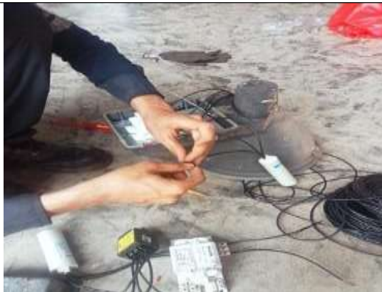
Gambar 3. 55 lampu Fire station 5
