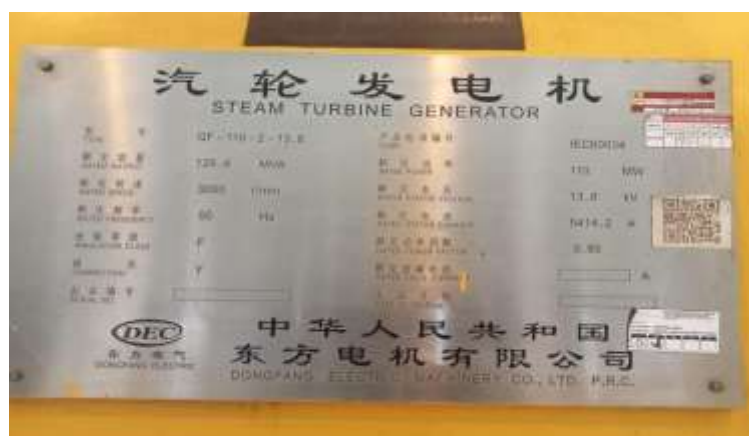
Gambar 4. 2 Nameplate Generator PLTU Tenayan
