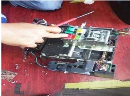
Gambar 3. 28 Repair Breaker C02 B
