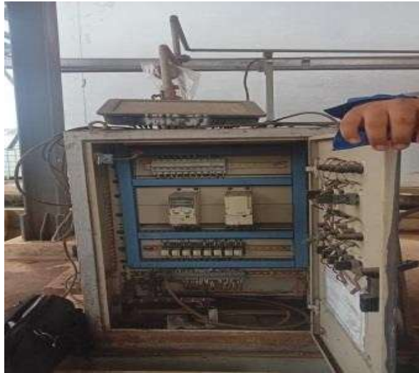
Gambar 3. 24 penggantian selector star Fly Ash
