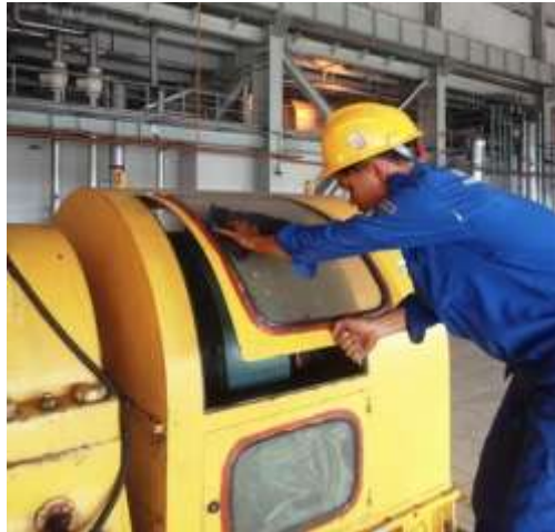
Gambar 4. 16 Membuka cover exciter
