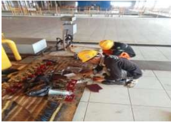
Gambar 3. 89 melakukan cleaning holder carbon brush
