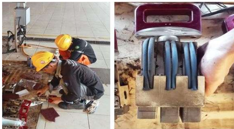
Gambar 4. 19 Cleaning Holder dan Carbon Brush
