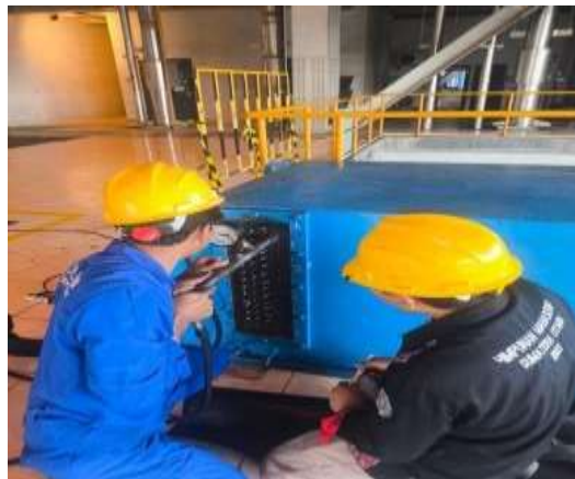
Gambar 3. 78 repair cooler motor Boiler Feed Pump 1 A
