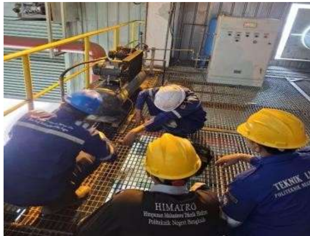
Gambar 3. 18 penambahan oil compresor
