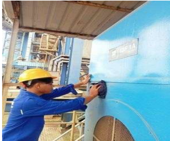
Gambar 3. 22 Preventive Maintenance Id Fan
