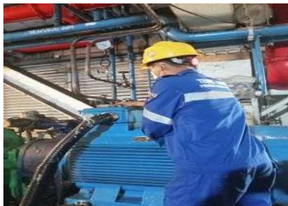
Gambar 3. 29 pemasangan coupling motor EX Close Cycle Water Pump
