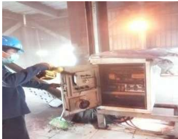
Gambar 3. 47 cleaning panel lokal vibrating screen
