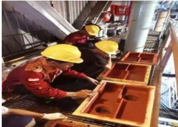
Gambar 3. 48 cleaning tutup cooler generator unit 2
