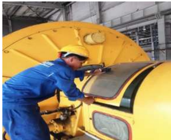
Gambar 3. 97 Gambar PM generator
