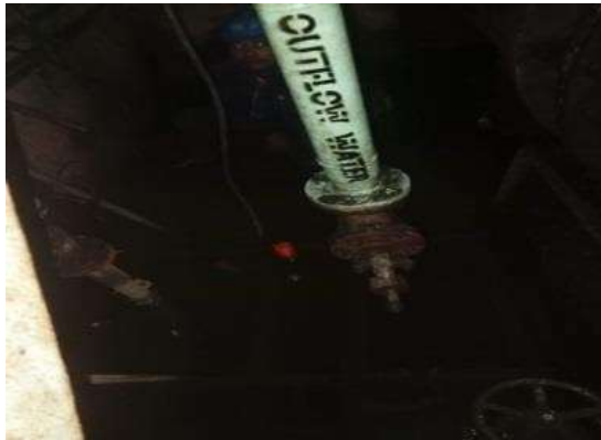
Gambar 3. 12 pemasangan level swith
