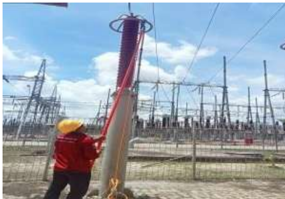
Gambar 3. 51 pengelepasan grounding trafo step up unit 1
