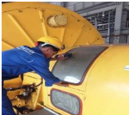
Gambar 4. 23 Proses menutup cavor exiter
