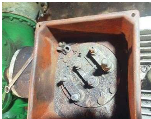
Gambar 3. 13 pengecekan hospot terminal motor (OCCWP)
