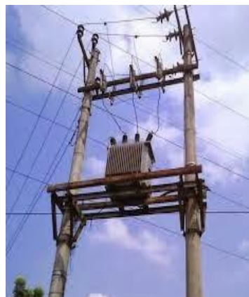
Gambar 3.3.5 Trafo distribusi
