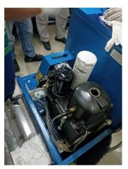
Gambar 3.42 Compressor Instrumen Air
