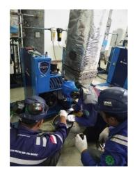
Gambar 3.39 Compressor Air Instrumen
