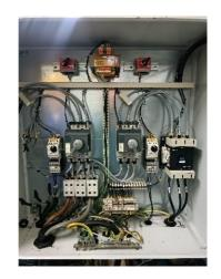
Gambar 3.27 Panel Kontrol Compressor Starting
