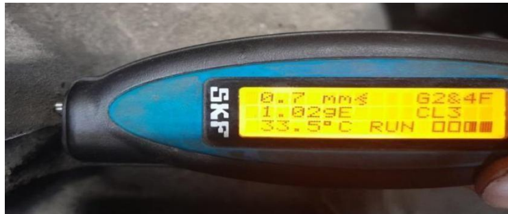
Gambar 4. 6:Pengecekan Vibrasi Bearing Sumber : PT.pacific indopalm industries
