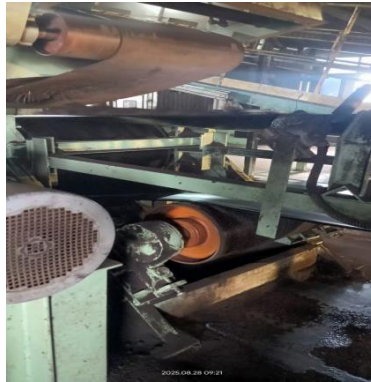
Gambar 4. 8 Tensioning Device (Sumber : Dokumentasi PT. Power Plant )
