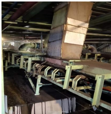
Gambar 4. 11 Safety Equipment (Sumber : Dokumentasi PT. Power Plant)
