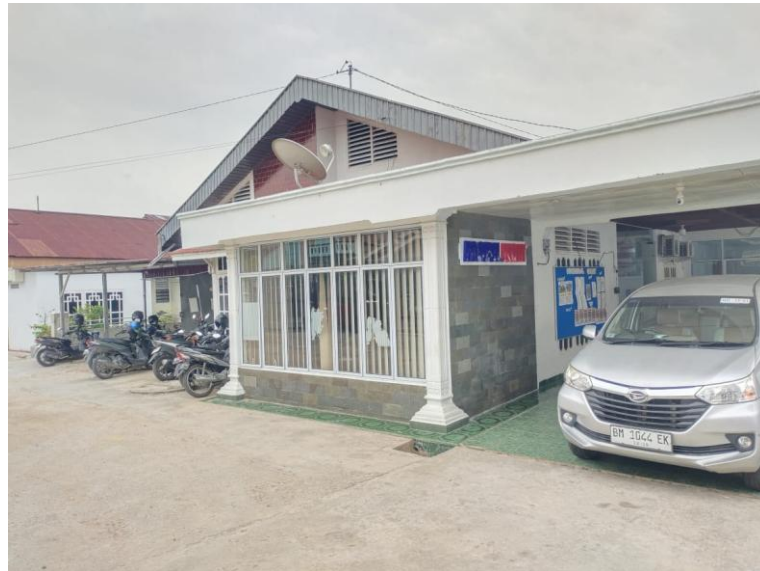
Gambar 2.1 Kantor PT Mobilkom Telekomindo Duri
