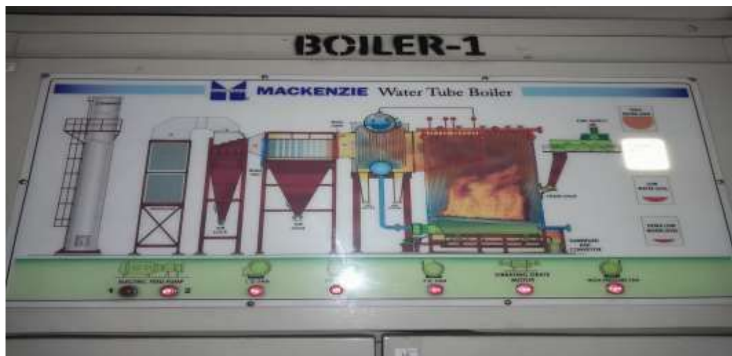
Gambar 4.2 sistim kerja Mackenzie boiler 2x20T/H
