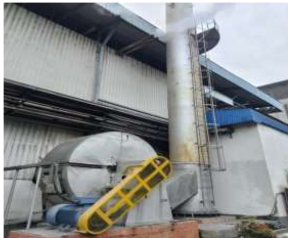
Gambar 4.4 induced draft fan (ID FAN)
