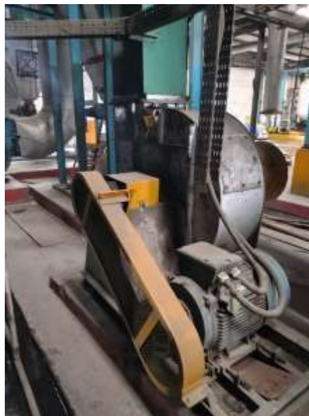
Gambar 4.5 secondary air fan
