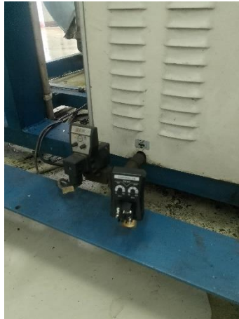
Gambar 3. 65 Replace auto drain valve
