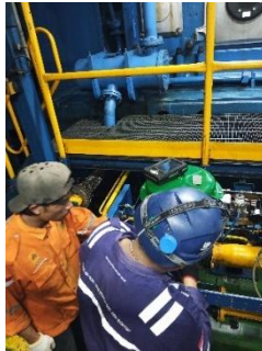
Gambar 3. 36 Gas control valve
