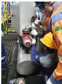
Gambar 3. 20 Motor Preheater
