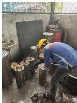
Gambar 3. 17 Filter booster
